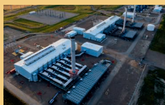
Pioneer Gen. Station Williston, N.D. • 2013 822 MW • Nat. Gas
