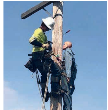
LREA's safety training program includes pole top rescue drills.
